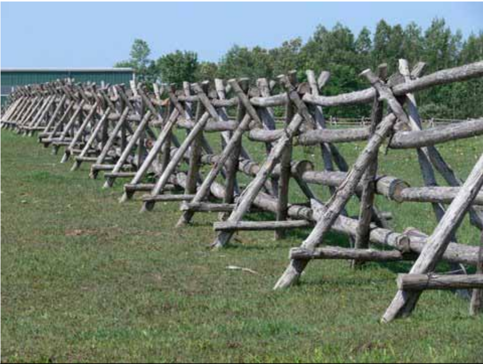
Patent or Bolton fence made with poles or split rails, supported at each end by a wired triangular support made of three pickets. This design represents the most sophisticated design of split rail fences, and is most frequently found in Eastern Ontario
