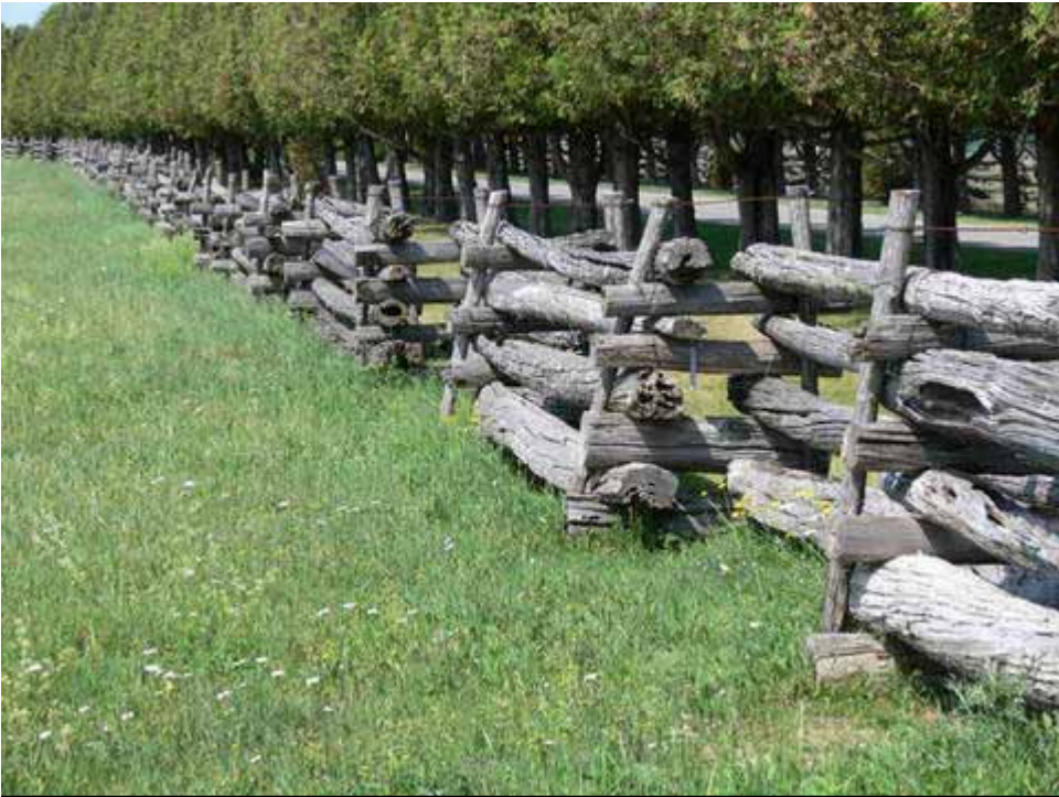
Log or bunk fence made with large logs, 12-16 feet long, spaced by short lengths of logs called bunks. Logs are in line, stabilized by small posts. In this design the logs are clamped by a bunk retainer.
