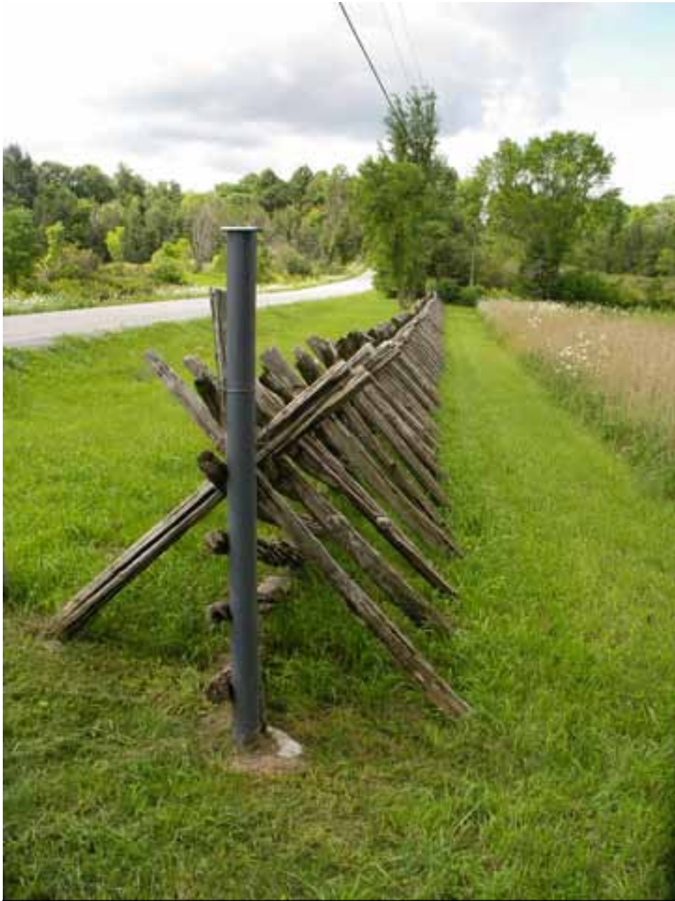
Indian or sheep fence made with poles or split rails, 12 feet long, one end resting on two pickets in an inverted "V", the other on the ground. It may be made with the pickets dug into the ground without wire, or with wire .
