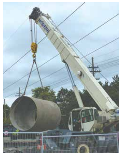
A tower foundation ready for dropping into its hole
