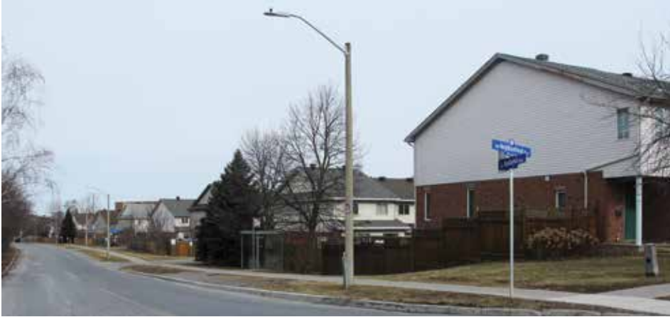
2004 – Townhomes were built by Claridge off Rolland Avenue. The streets were named Sienna Private and Santa Cruz Private.
