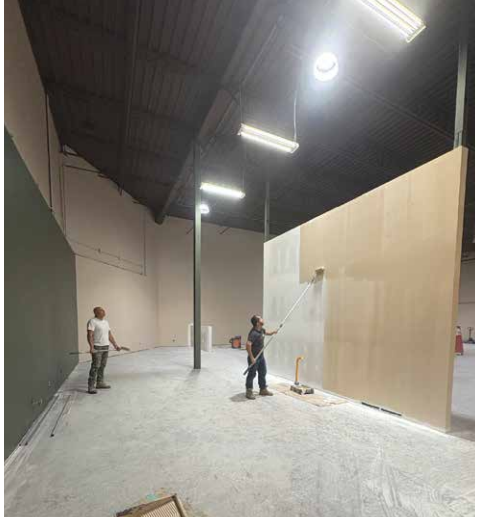
The wonderful progress at Matthew House.
